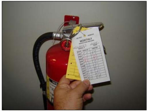
Figure 34. Monthly fire extinguisher tag inspection record
