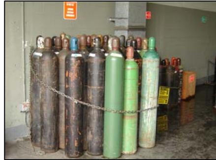
**Figure 20. Cylinders will be secured in carts or storage areas with a strap above its center of gravity**
