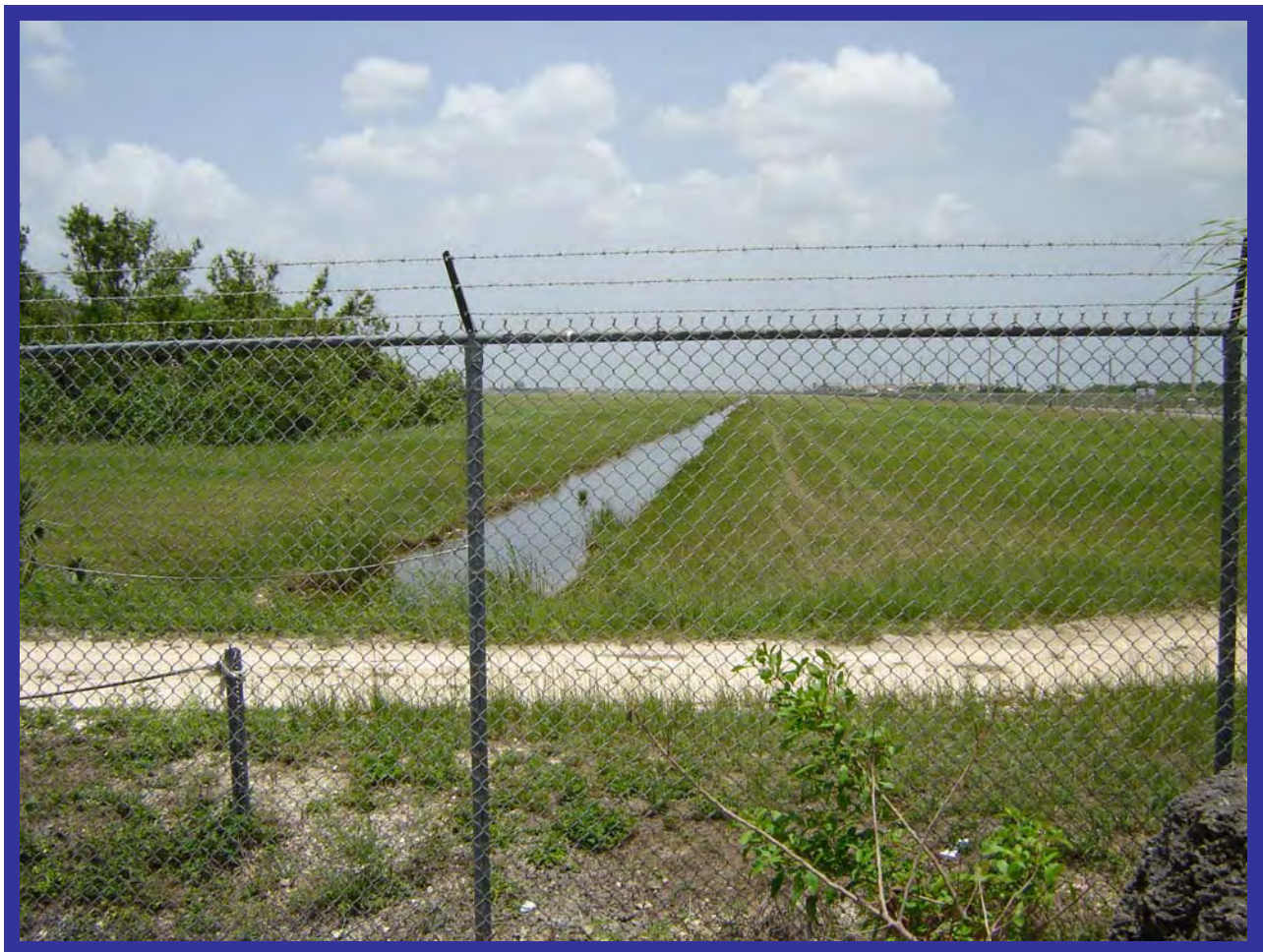
FLUCFCS Code 510 – Canal
