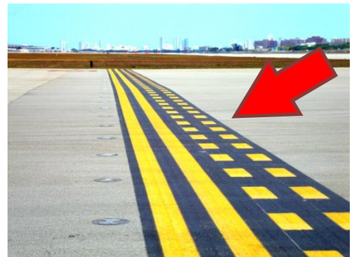
Figure 4, Runway Hold Position Marking
