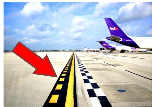
Figure 1, Non-Movement Area Boundary marking shown with roadway checker edge marking.
